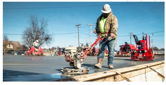
The compact weight and size of the Pro424E walk-behind trowel makes this easy to use for tight areas. This walker is great for edging against walls, pipes and other obstructions, and will fit easily through doorways. This unique compact walker, with the collapsable folding handle, allows for easy transportation.
